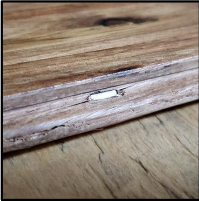
Cleat properly driven and no splitting
