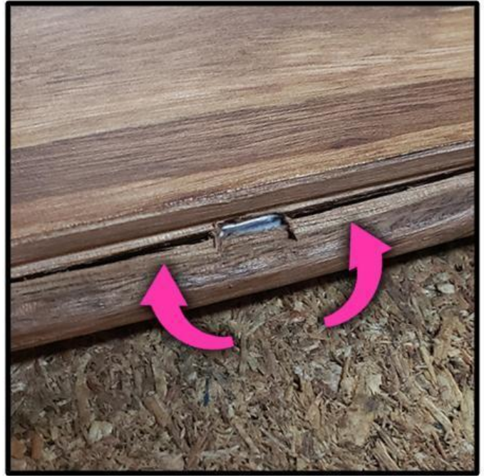
Cleat properly driven and some splitting
